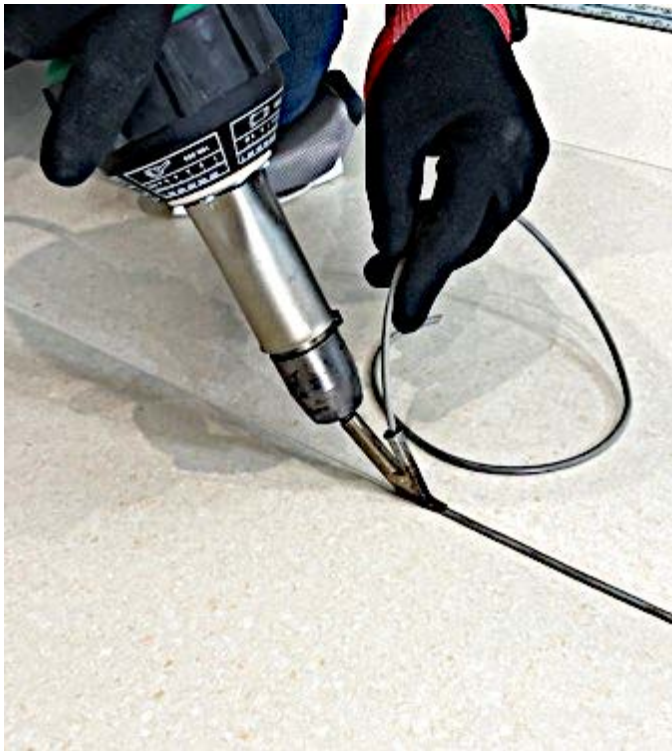
Figure 23 - Heat welding
