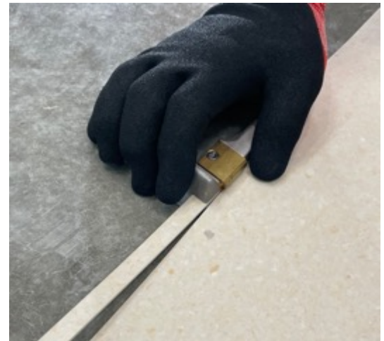
Figure 15 – Trim the factory selvage from the edge of the roll for proper seam construction.
