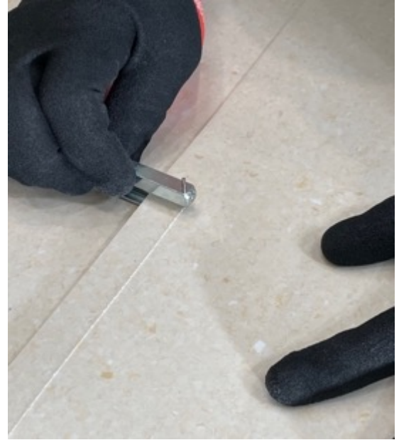
Figure 17 - Depicts the recess scribe scoring the top sheet of flooring.
