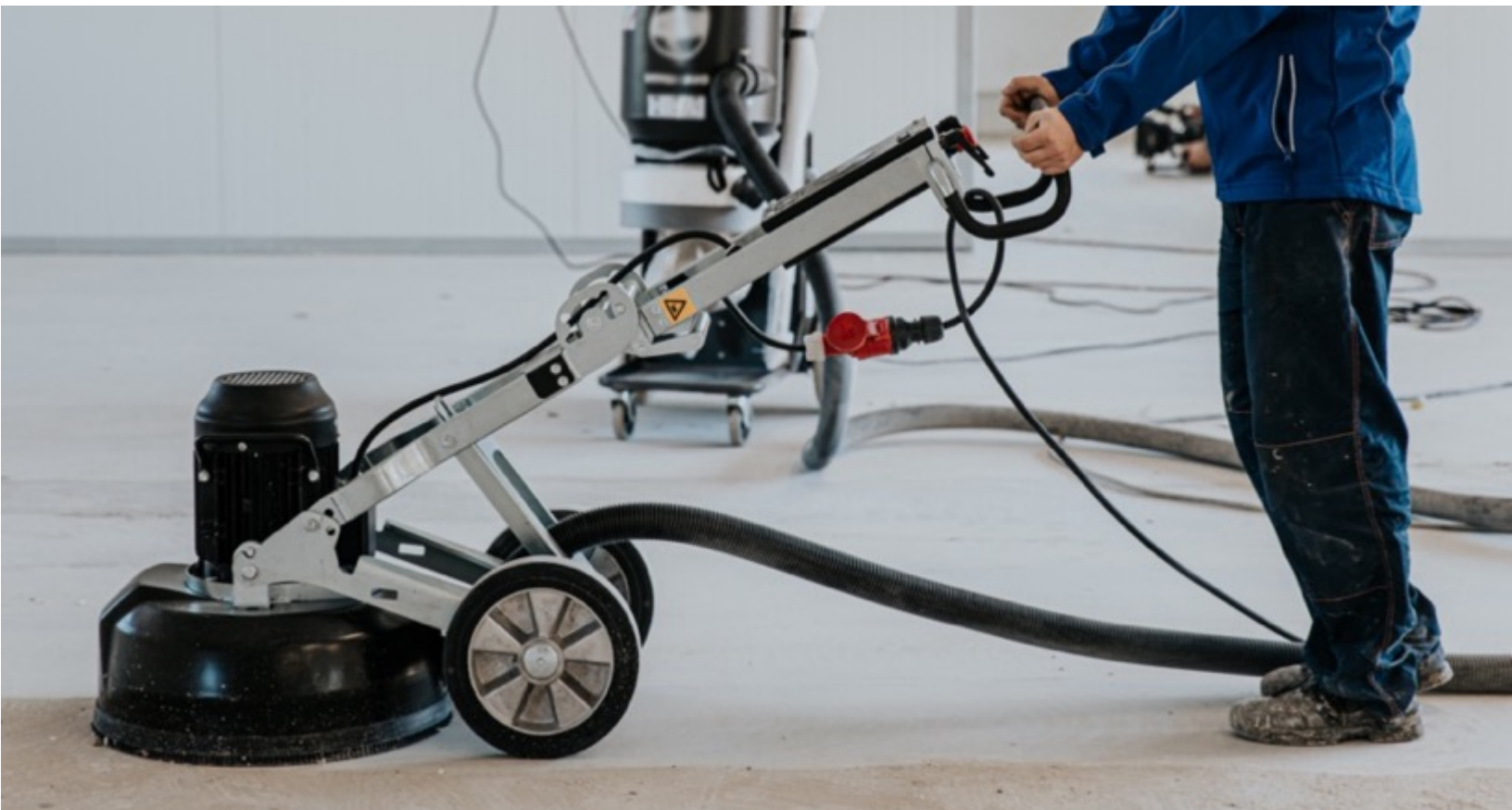
Figure 9 - Contaminate removal is a critical part of a successful installation.
