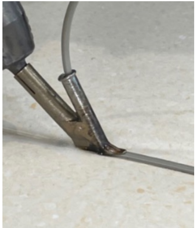
Figure 23 - Close up of heat welding
