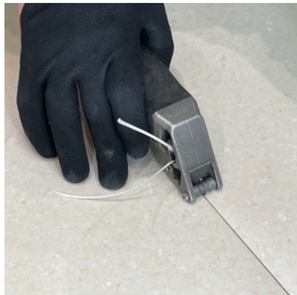
Figure 18 – Depicts the grooving of a seam using a push-type groover.
