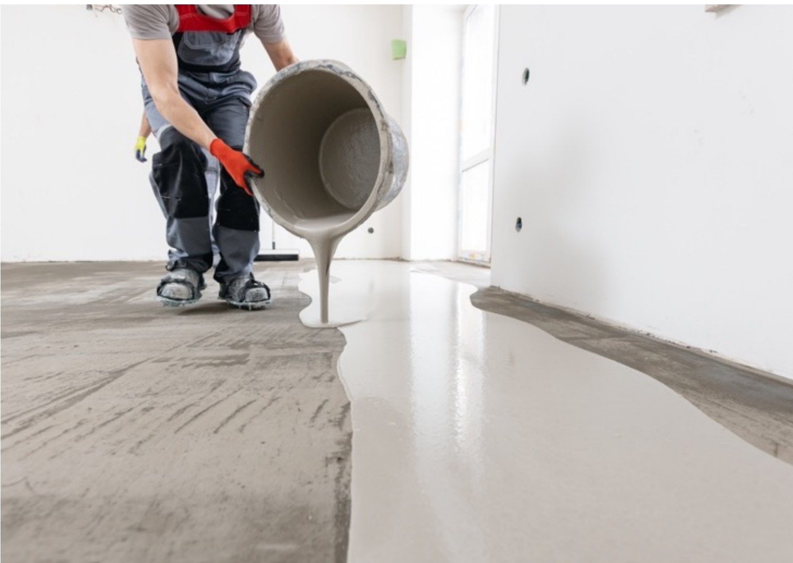
Figure 10 - Always perform floor preparation in accordance with ancillary manufacturer’s instructions.
