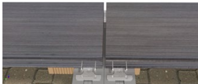
18. Installation of two battens between headers with a clip for each slat.
