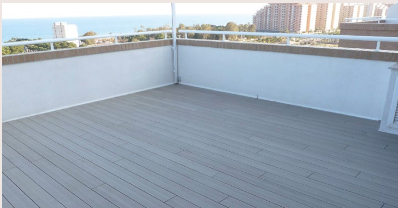
24. Assembled deck with invisible joint.
