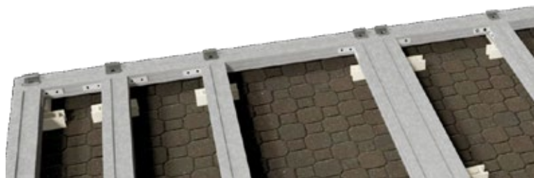
33. Starting the installation with the initial clip.
