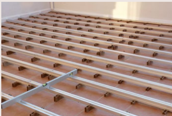
22. Batten installation for an invisible joint.
