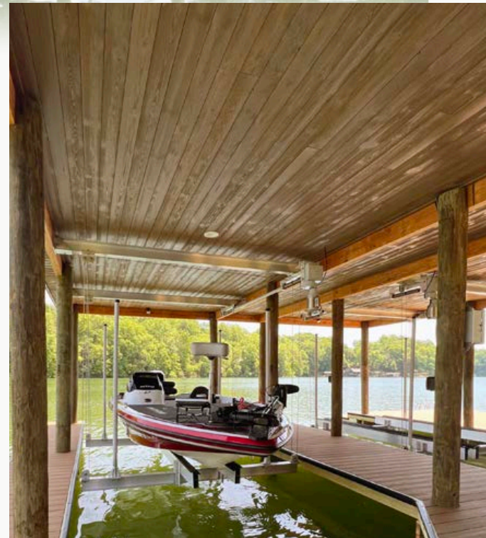
Knoxville, TN Design-Build: Dock & Deck
