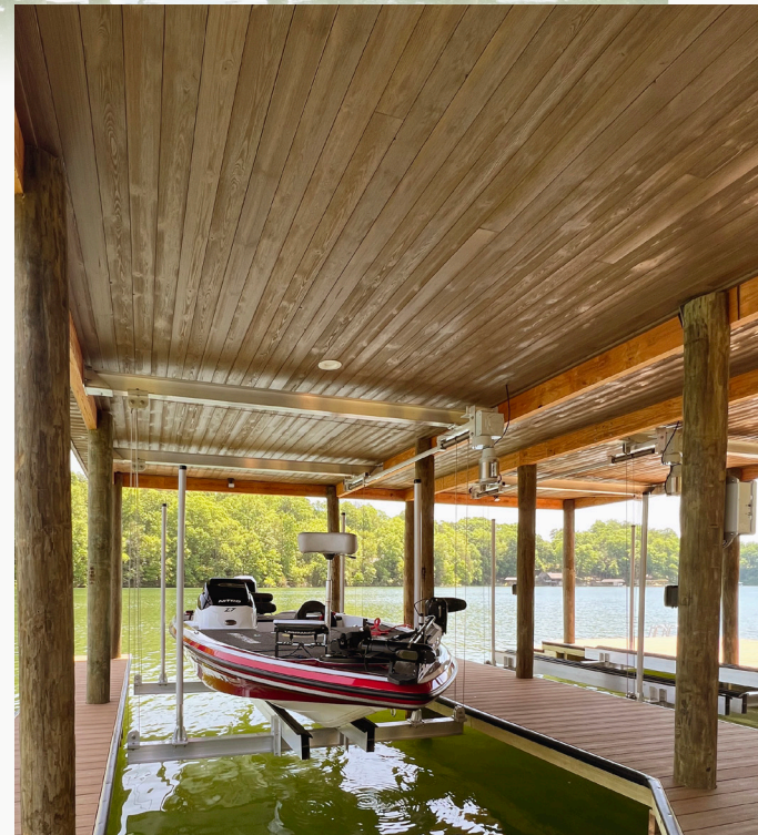
Knoxville, TN Design-Build: Dock & Deck
