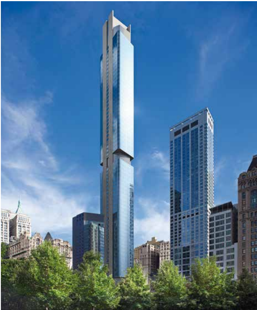
125 Greenwich Street , New York, USA design / Rafael Vinoly Architects PC
