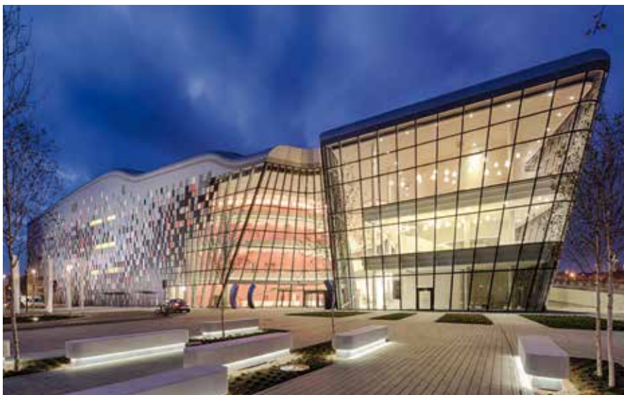
ICE Congress Centre , Cracow, Poland design / Ingarden & Ewý Architekci, Arata Isozaki & Associates
