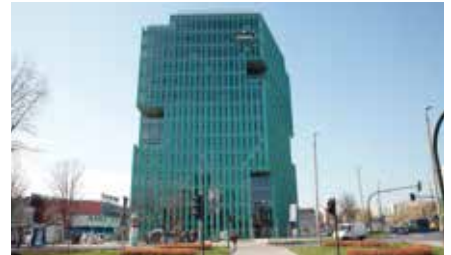
Alma Tower, Cracow - LEED PLATINUM
