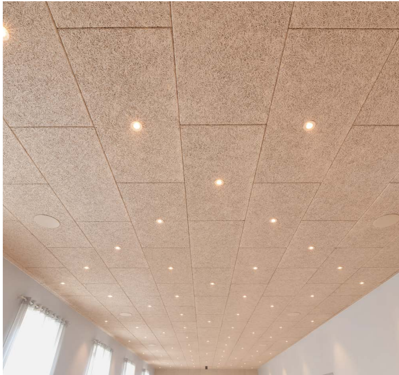
Recessed lights installed into the ceiling
