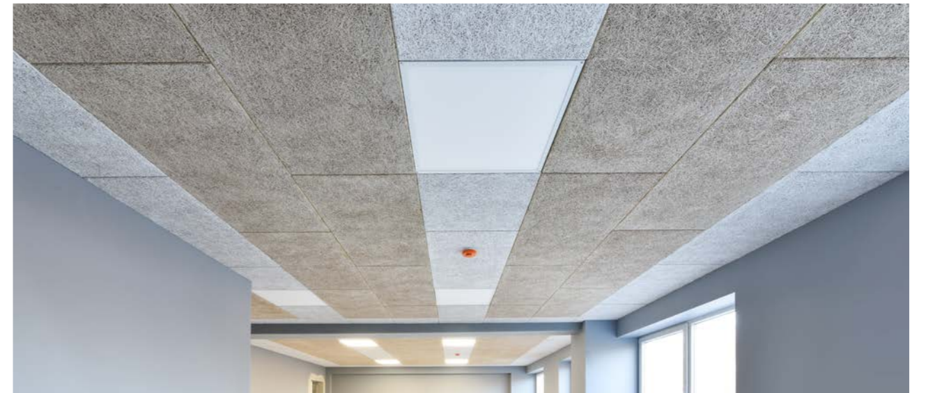
T-type profile frame, P0G edge profile, 25 mm CEWOOD Acoustic panel.
