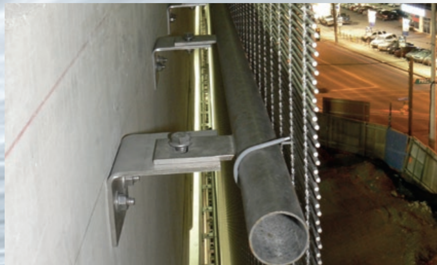
Intermediate mounting: round tube and wire connectors.
