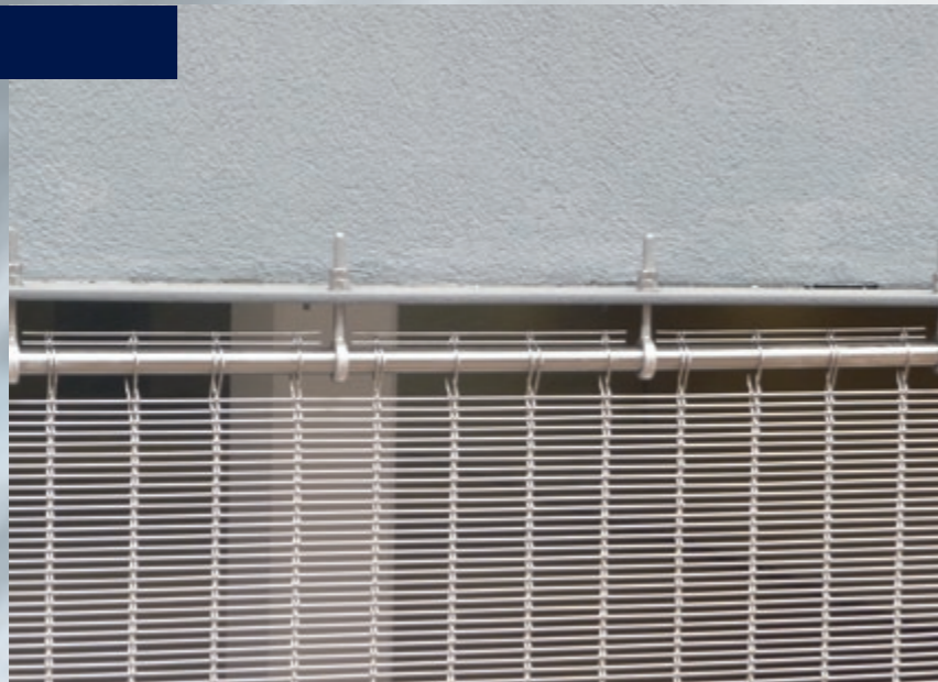
Top mounting: round bar with eyebolts.
