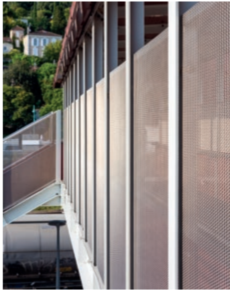
Semi-transparent railing infill made of EGLA-DUO 4222. Railroad station Agen, France.
