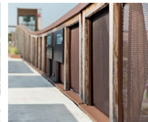
Painted with brown textured lacquer. Pedestrian bridge Lisieux, France, DOKA-MONO 1421.
