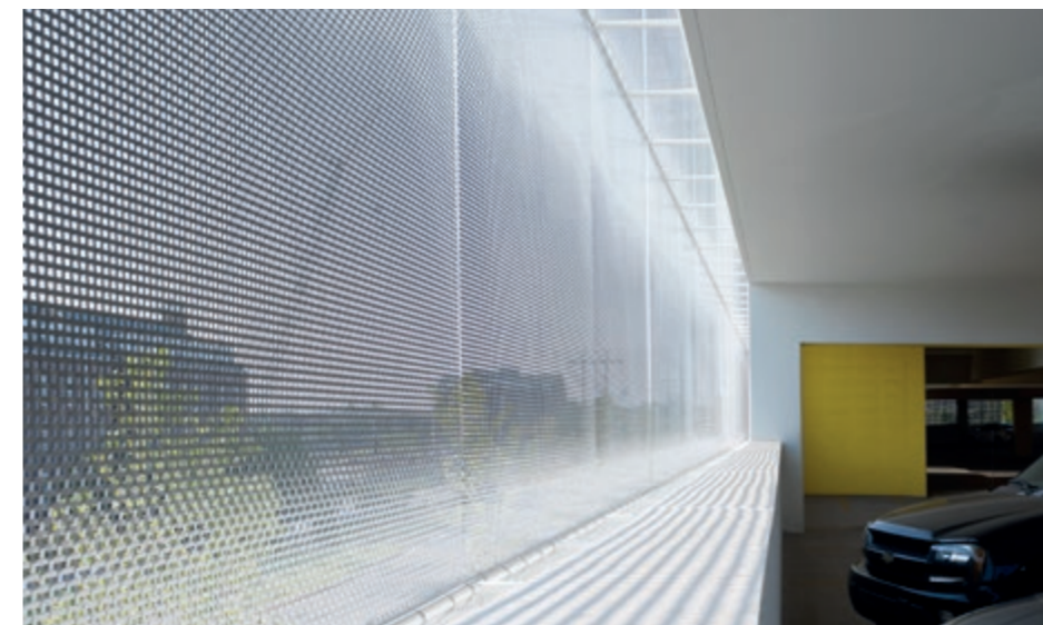
Sun protection with a good view from inside. Car park, Chesapeake, Oklahoma, USA, LARGO-PLONUS 2022.
