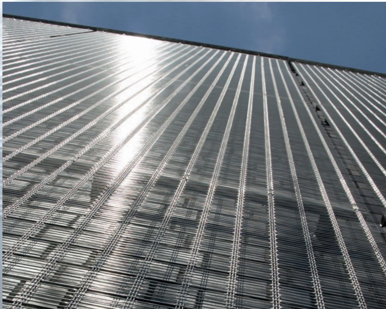
Architectural mesh can be tensioned vertically over several storeys. Load-bearing substructures are only required on the upper and lower face. Facade cladding DOGLA-TRIO 1032, Germany.
