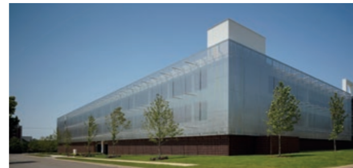
View during the day. Stainless steel mesh LARGO-PLENUS 2022, Car Park Chesapeake, Oklahoma, USA.
