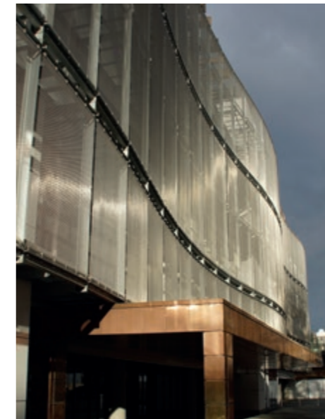
Wave-shaped facade cladding: Holland Park School, London, Great Britain, ECLA-MONO.
