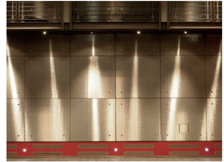
Architectural mesh MINIFLEX 8135 makes the walls of the proscenium at Luxembourg's Théâtre Municipal shine.
