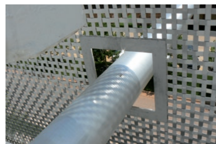
Cut-outs in mesh elements.
