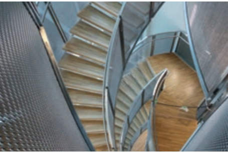
Wire mesh as stylish balustrade infill. St. Michael's Hospital, Toronto, Canada, EGLA-TWIN 4223.
