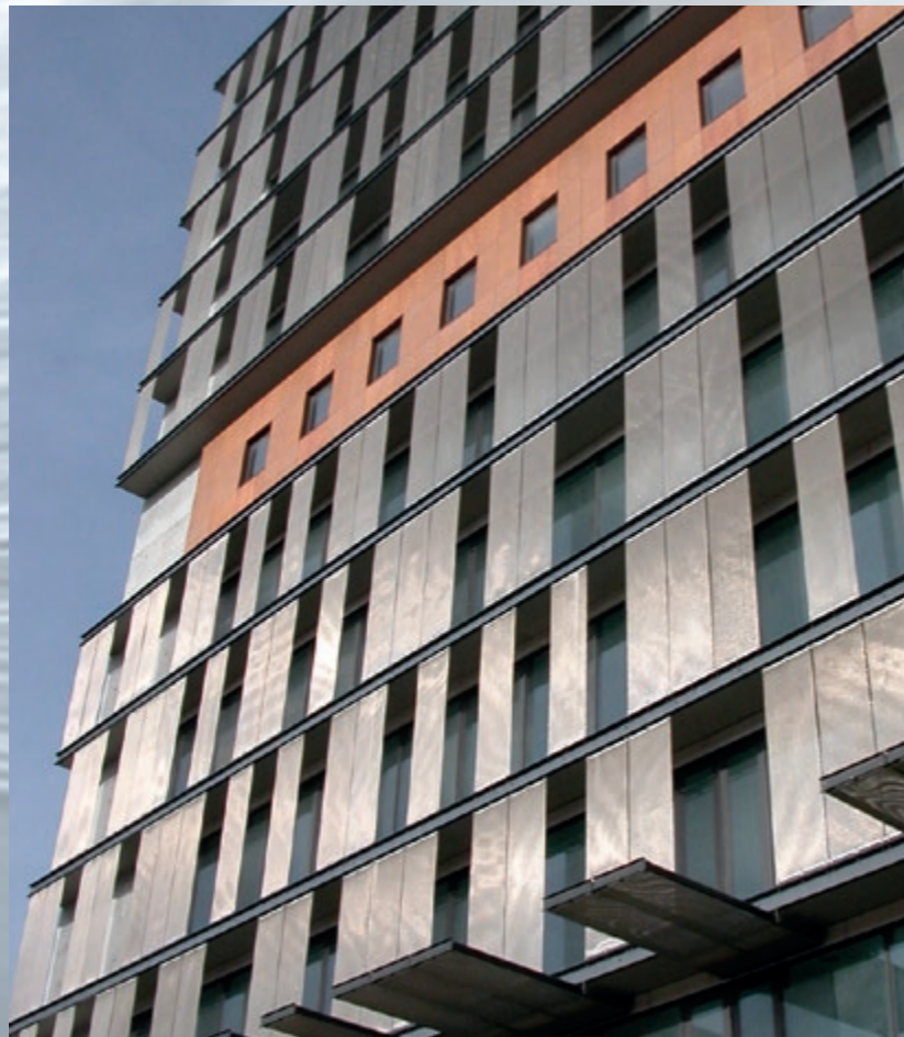
Transparent architectural mesh elements effectively combine sun protection with superb design possibilities. Sun protection facade, Lisbon, Portugal, ECLA-MONO 4391.
