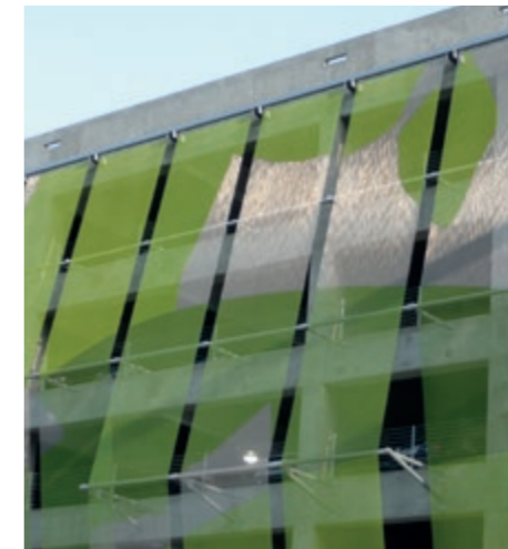
Partially painted mesh elements. Los Angeles Police Department, USA, EGLA-MONO 4832.
