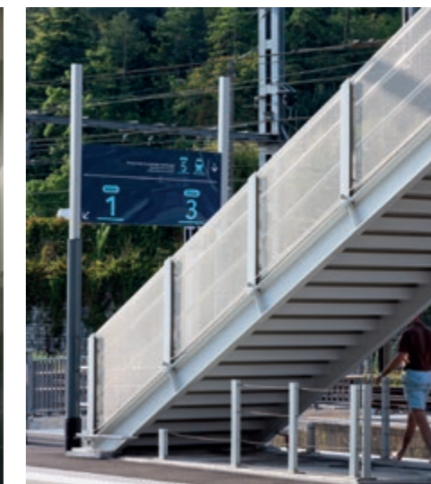
Bridge cladding at a train station made of stainless steel wire mesh EGLA-DUO.
