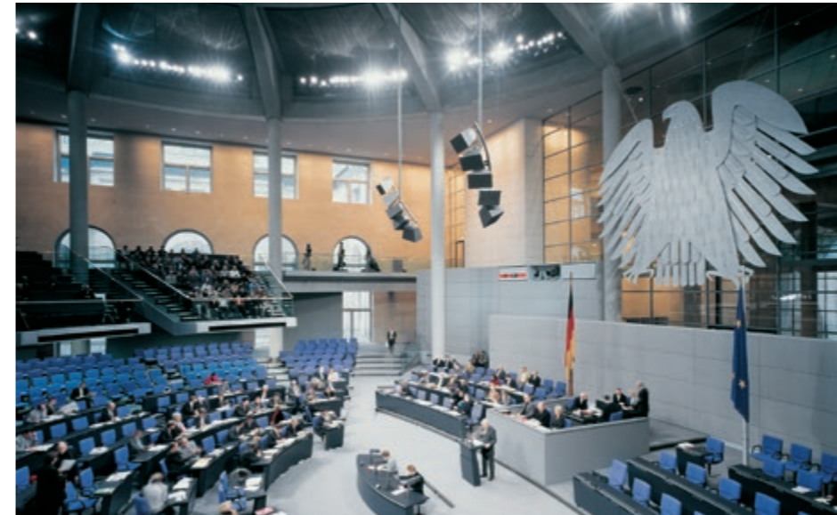
Modern acoustic fleece behind an elegant stainless-steel veil. Plenary Hall of the Reichstag building, Berlin, Germany, DOKA-MONO 1601.
