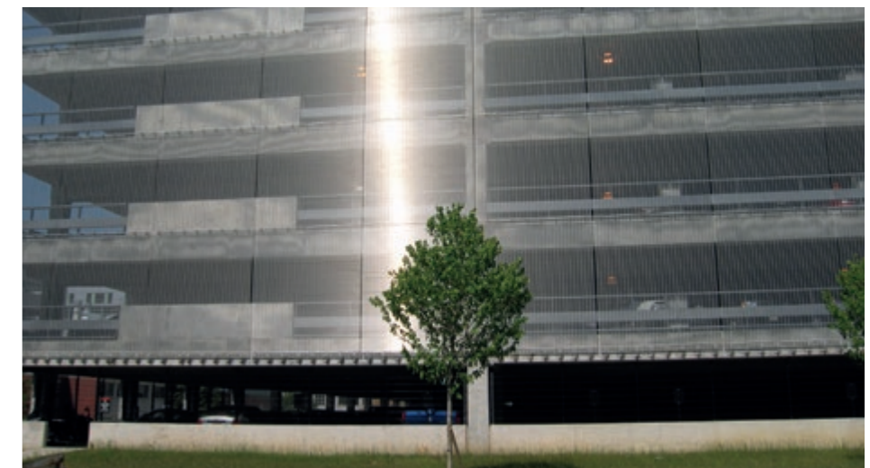
When interacting with sunlight, stainless-steel wire mesh gives facades an elegant, shimmering appearance. Car park cladding MULTI-BARRETTE 8301, Ohio, USA.
