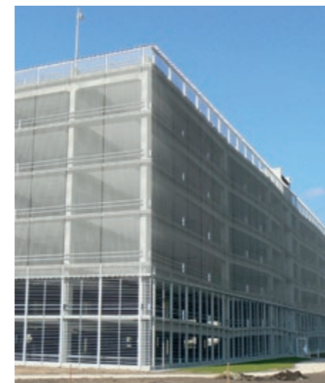
Facade cladding of a parking garage with the HAVER Architectural Mesh DOGLA-TRIO.
