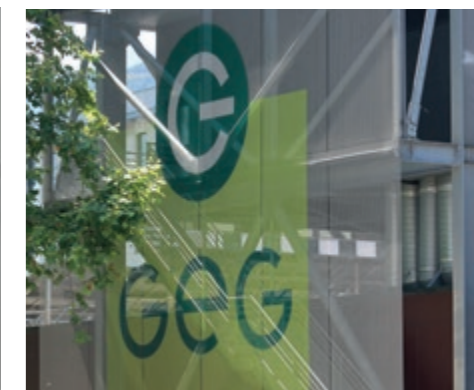
Painting DOKAWELL-MONO 3571, Gaz Electricité de Grenoble, France.
