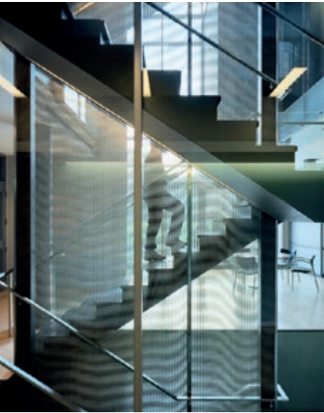
Stairwell cladding using two layers of architectural mesh to create the moiré effect. McGill University, Montreal, Canada.
