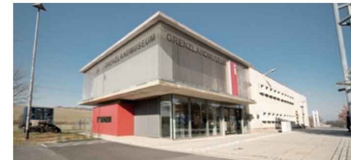
EGLA-TWIN 4313 wire mesh facade during the day. Eichsfeld Borderland Museum, Teistungen, Germany.
