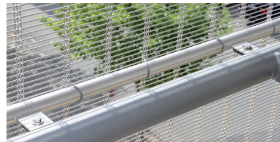
Intermediate mounting: round tube and wire connectors.
