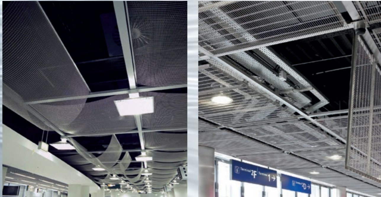
Adjustable mounting system for ceilings with sag.
