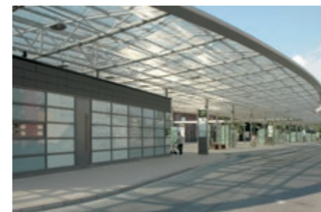
Wire mesh as sun protection. Herne Bus Station, Germany, DOKAWELL-MONO 8967.
