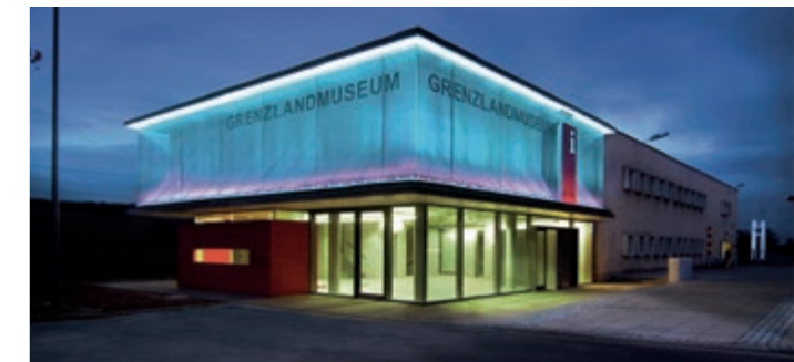
Night-time view with backlit wire mesh.
