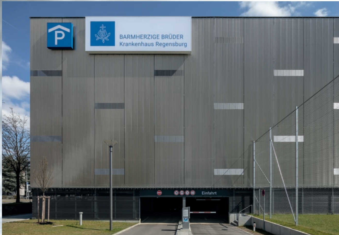
Closed but still transparent parking garage facade cladding made of the stainless wire mesh LARGO-TWIST 2051. Regensburg, Germany.
