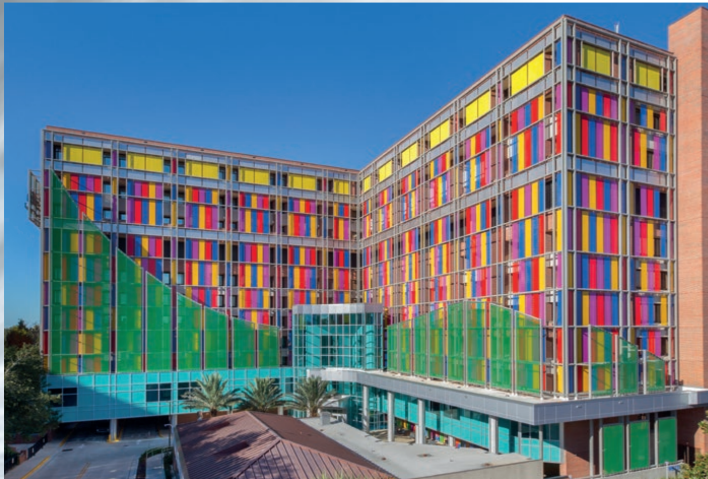
Colourful facade cladding of architectural wire mesh. Shands Children's Hospital, Gainesville, Florida, USA, LARGO-PLONUS 2022.
