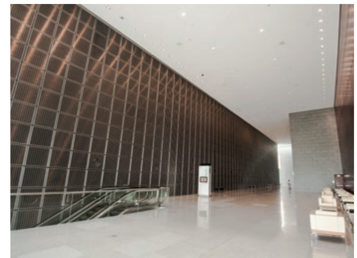
Wire mesh cassettes made of architectural mesh MULTI-BARRETTE 8123. Qatar National Convention Centre, Doha, Qatar.
