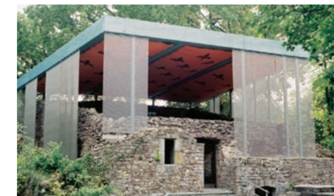
The semi-transparent stainless-steel mesh LARGO-NOVA 2017 encloses the existing building and ensures natural lighting. C&A Eco Store, Mainz, Germany.
