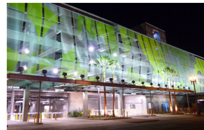
HAYER Architectural Mesh panels, partially painted. Parking garage Los Angeles Police Department, USA.
