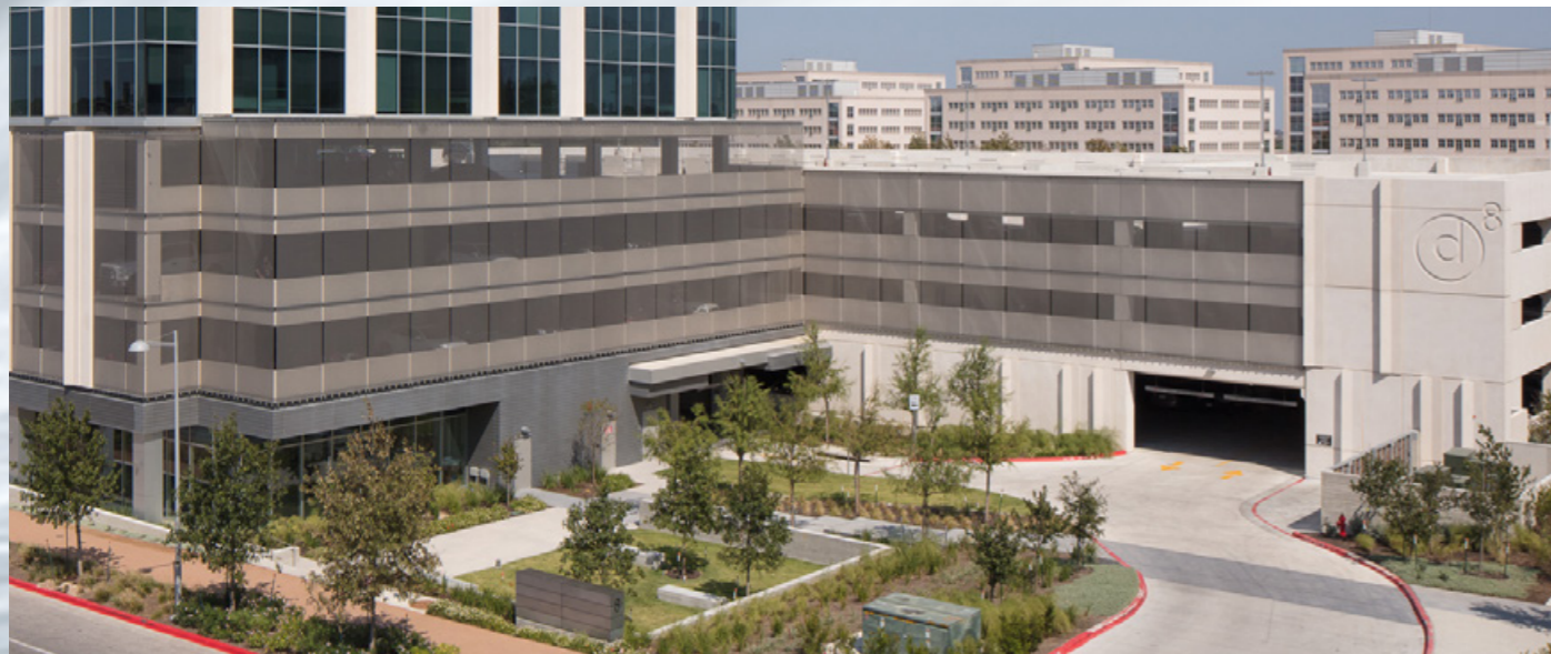
Semi-transparent facade cladding with HAYER Architectural Mesh. Car park Domain8, Austin, USA.
