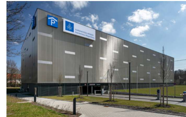
Large-scale wire mesh cladding with homogeneous appearance. Parking garage Barmherzige Brüder Hospital, Regensburg, Germany.
