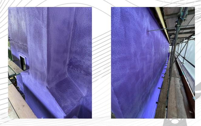
All external walls are air/smoke tight before external wall insulation is fitted.
