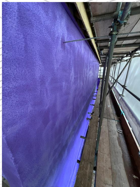
**All external walls are air/smoke tight before external wall insulation is fitted.**
