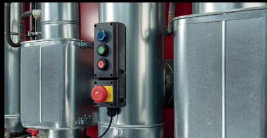
EX push button open-close (photo: R steel)
