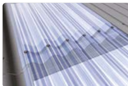
DETAIL OF OVERLAP Detail of overlapping components
