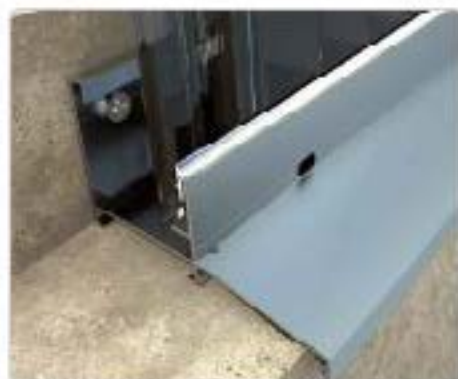
BASE PROFILE Detail of curtain wall, insertion in base profile
