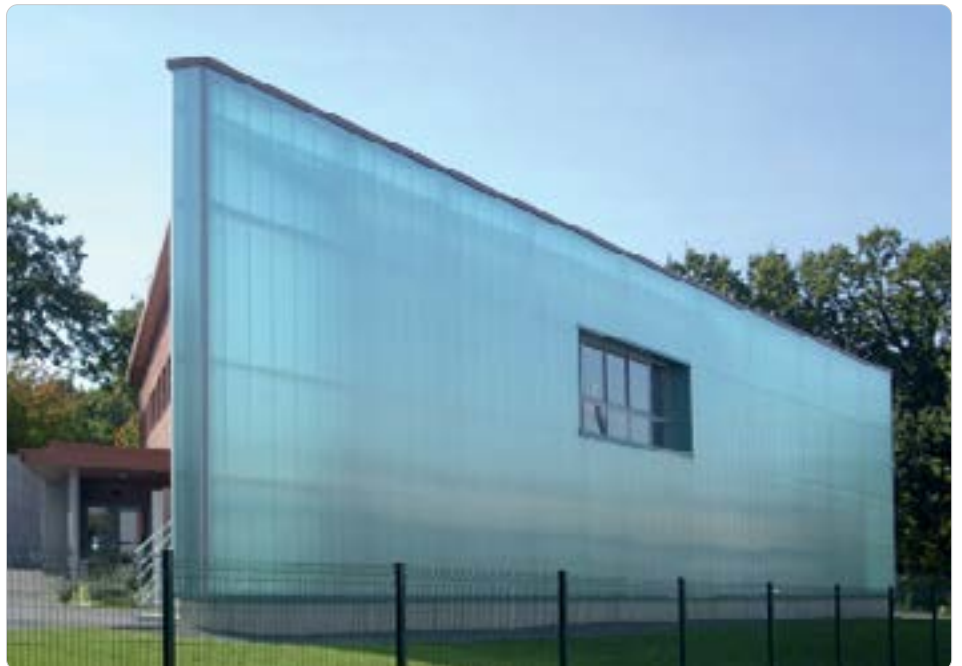
TRANSLUCENT CURTAIN WALLS Realization vertical translucent curtain walls
