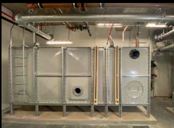
INDOOR TANK WITH PEDESTAL STEEL FOOTING OPTION
