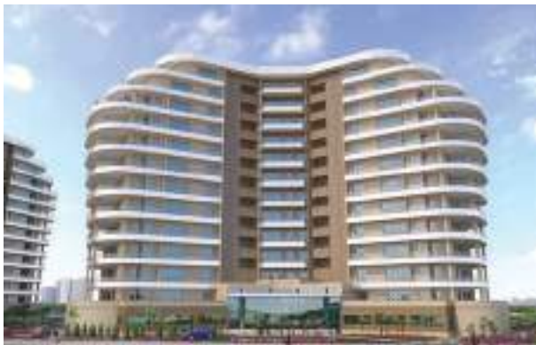
● PARSIS APARTMENT BUILDING PROJECT / IRAN
