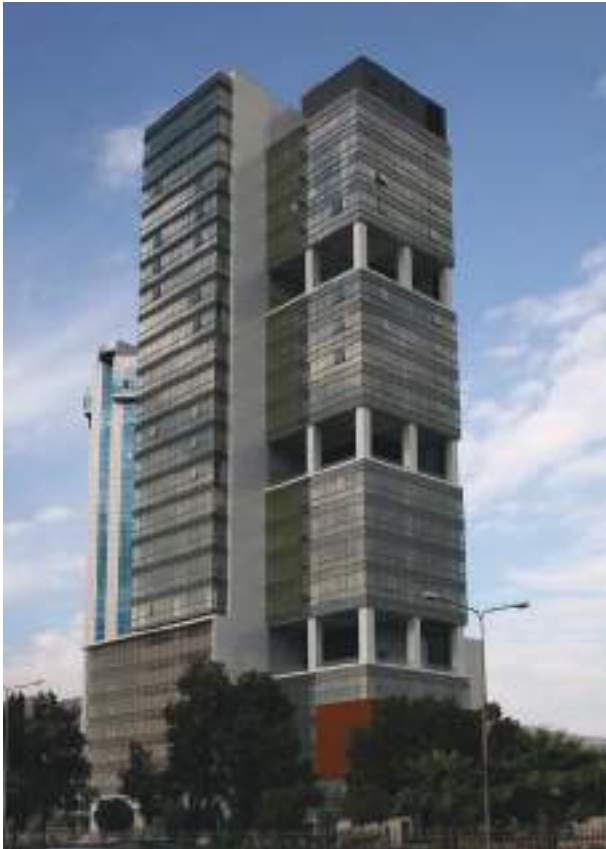
● MEGAPOL TOWER / IZMIR, TURKEY
