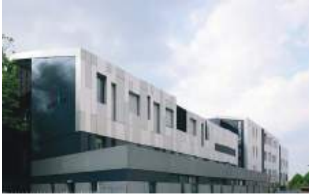
● DEMATHIEU & BRAD HEALTH CENTER / GENNEVILLIERS, FRANCE
