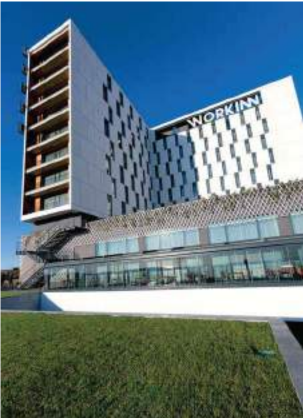
● WORK INN HOTEL / ISTANBUL, TURKEY
