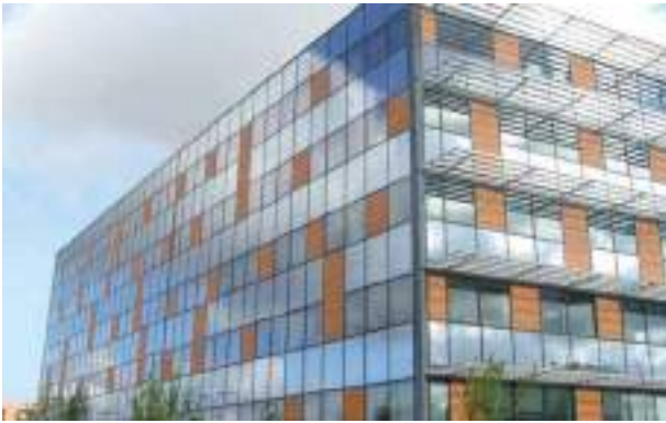
● SOGEA TP1 & TP2 - VINCI MAIN HQ / FRANCE
