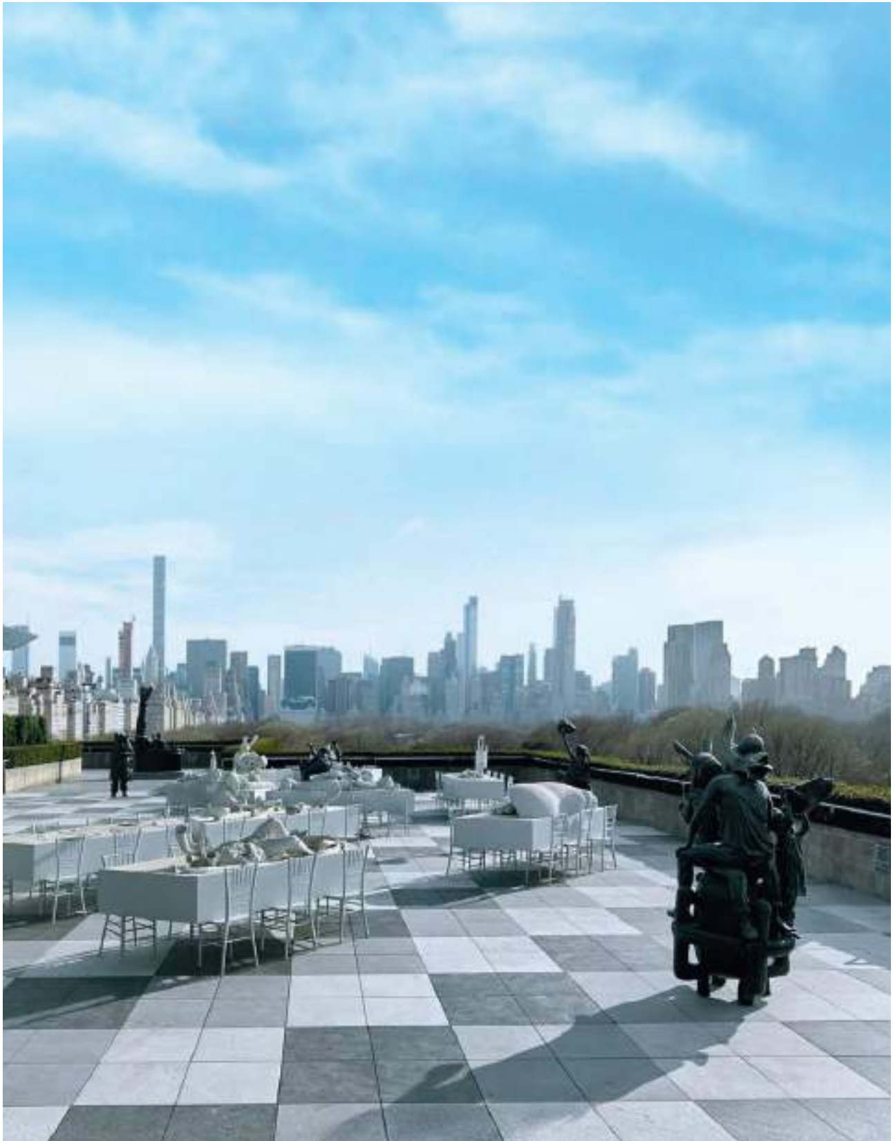
Metropolitan Museum of Art – Temporary Roof Garden New York, U.S.A. Pedestal System – Eterno SE
