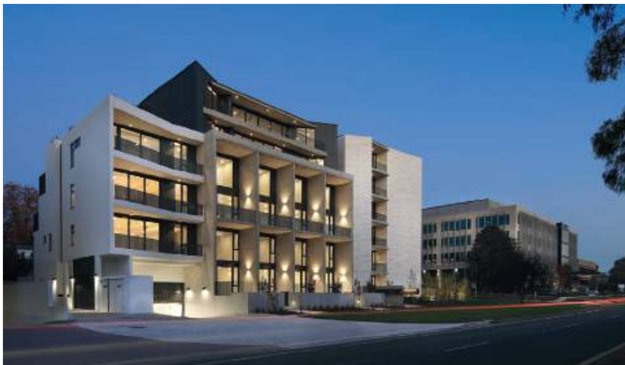
Dominion Apartments - Rooftop, terrazze e aree esterne Canberra, Australia Pedestal System - New Maxi NM
