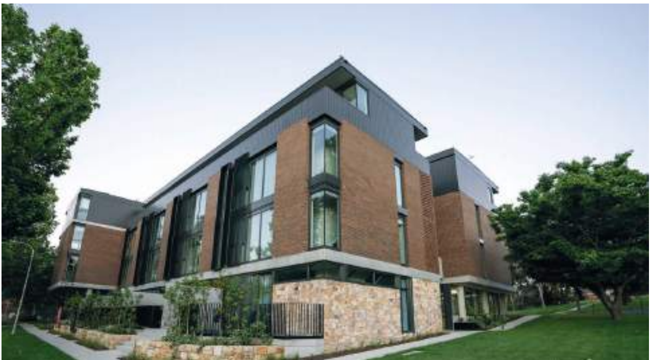
MICA (Middle of Campbell) – Rooftop, terrazze e aree esterne Campbell, Australia Pedestal System – New Maxi NM
