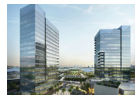
Shenzhen Exhibition Bay East City Property type: Apartments Developer: Shenzhen zhaohua Number of residences: 800
