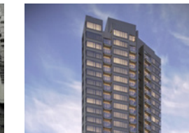
18 Junction Road Property type: Residential/business building Developer: SINO Group Number of residences: 80
