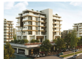
Livin' Izmir Property type: Residential Developer: Cengiz Construction Number of residences: 363
