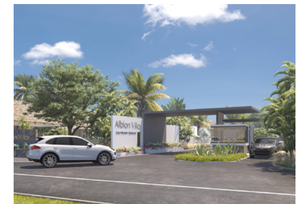
West Coast Albion – Mauritius Property type: Residential Developer: Exclusive Albion Villas Ltd Number of residences: 39
