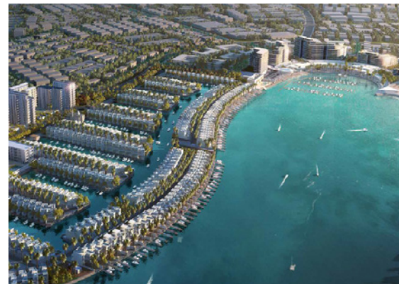
Al Naseem Phase 1 Property type: Residential Developer: Diyar Al Muharraq Number of residences: 200
