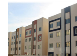
BAWAB Buildings Property type: Residential Developer: BAWAB Contracting Number of residences: 150
