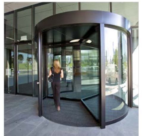
800 Collins Street, Docklands
