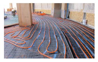
Watts Radiant® and SunTouch snow melting systems
