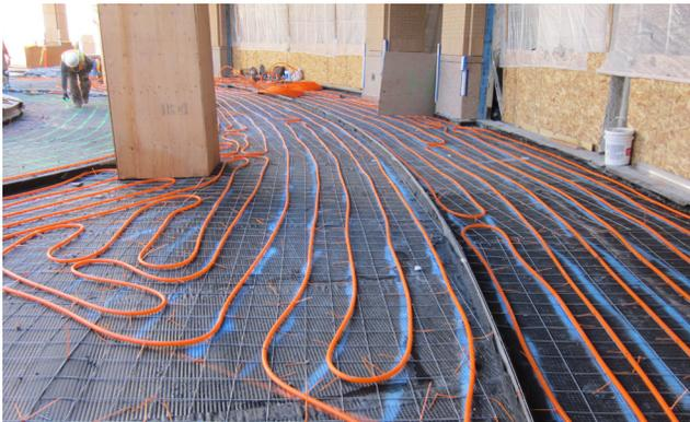
Watts Radiant® and SunTouch snow melting systems
