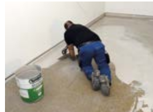
Application of main coat
