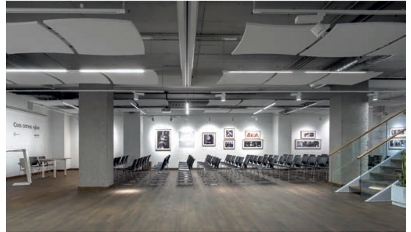
Hanging luminaires can provide accent or general lighting, allowing spaces to be categorised.
