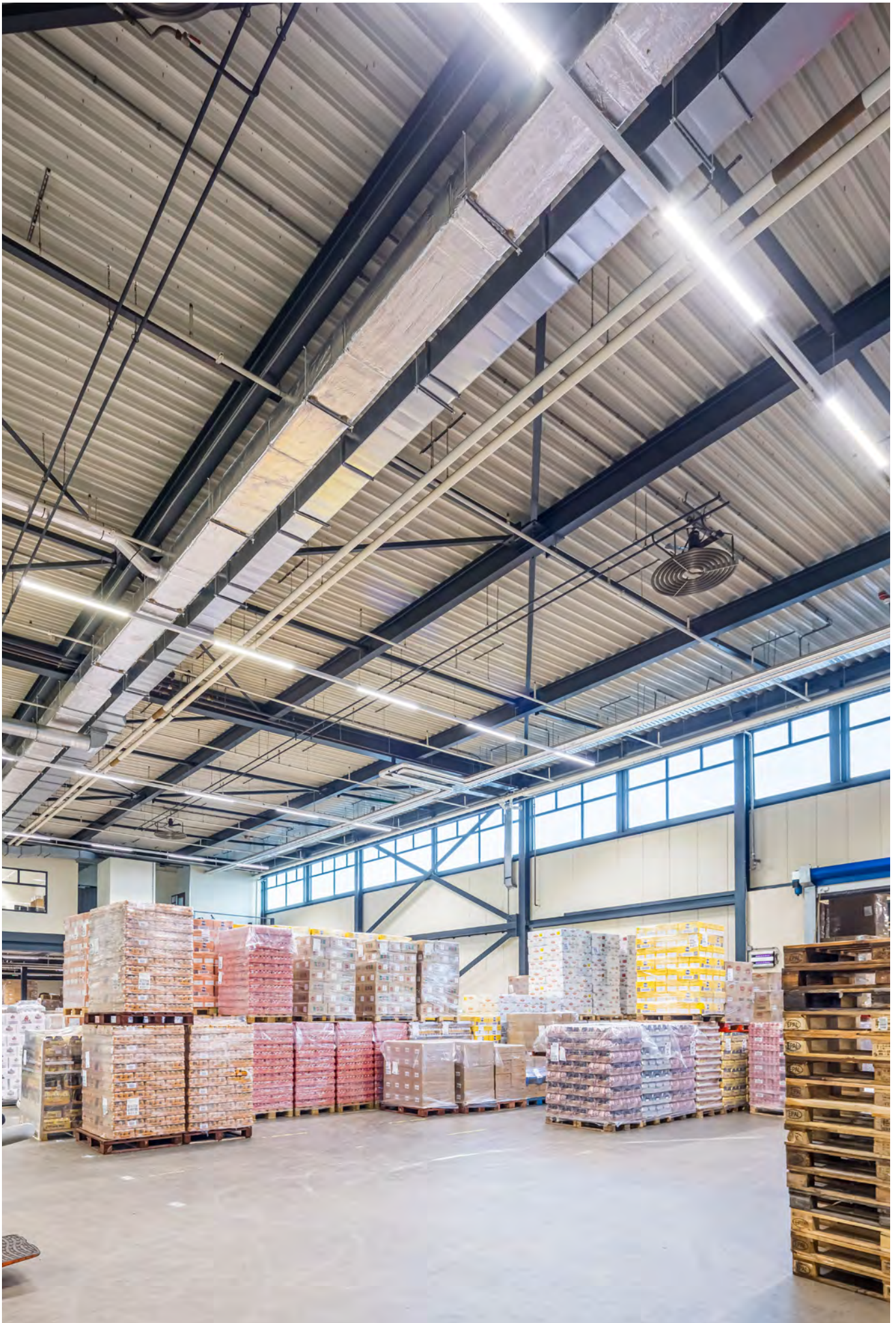
Unidex warehouse - De Zilk - Netherlands
