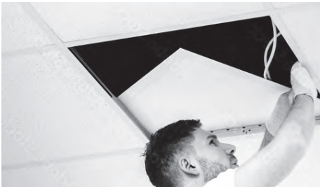
Modernisation work – this LED lighting series is especially suitable for 1:1 replacement.
