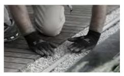
For outdoor applications, provide drainage gravel for at least 300 mm additional to the appliance or a suitable drainage system
