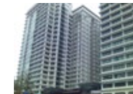
North Point Condominium
