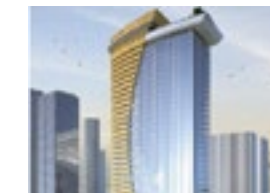
Al Barooq Tower Property type: Residential Developer: KBM Builders Number of residences: 500
