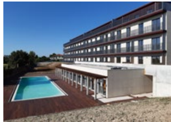
Asprela Gardens Property type: Residential Developer: JMC-Investimentos Imobiliários, Lda. Number of residences: 111
