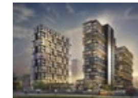
Se Retro 9 Property type: Residential Developer: Aşçıoğlu Construction Number of residences: 218
