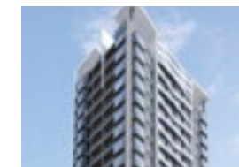
YO HO City Centre Property type: Residential Developer: Hin Lok Real Estates Company Ltd Number of residences: 237
