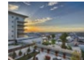
Wave Muscat Property type: Residential Developer: Al Mouj Muscat Number of residences: 240
