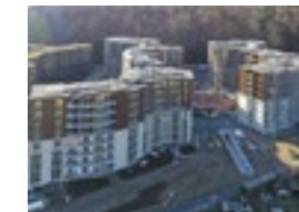
Neubauwohnsiedlung Guggach II Zurich Property type: Residential General Contractor: HRS Real Estate AG Number of residences: 257
