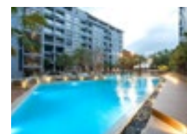
Citygate Phuket Property type: Premium residential in Thailand's top beach destination Developer: Citygate Exclusive Development Number of residences: 388
