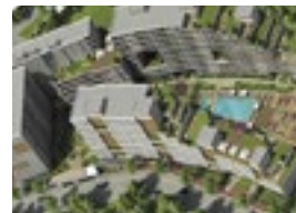
Selective Port Property type: Residential Developer: Alper Construction Number of residences: 315
