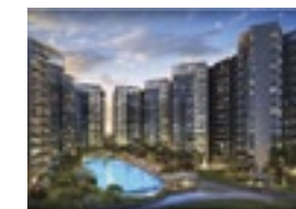
The Scala Property type: Residential Developer: UOL Group Limited Number of residences: 570
