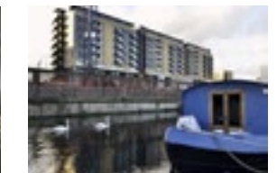
Suttons Wharf North Property type: Residential Developer: Hollybrook Number of residences: 450
