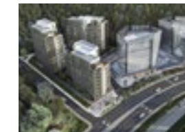
Vadi Kuru Property type: Residential Developer: Invest Construction Number of residences: 288
