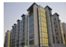
Paramount Tower Property type: Residential Developer: Qatar Airways Number of residences: 415
