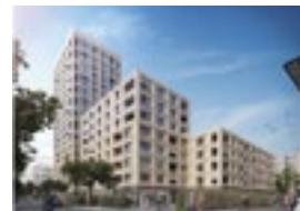
Labitzke Areal, Zurich Property type: Residential Developer: Mobimo AG Number of residences: 277
