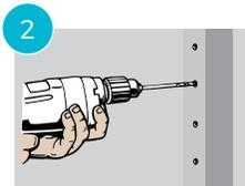
Drill 5/16" holes in one End Post for the Threaded Terminal Fitting, 3/8" holes in the other End Post for the Quick-Connect® Fitting, and 1/4" holes in all other Posts.
