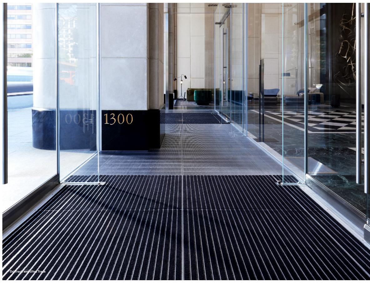
Architectural grilles enhance a property's aesthetics while providing performance characteristics- including promoting positive indoor air quality, removing moisture and debris and withstanding high foot traffic and heavy rolling loads.
