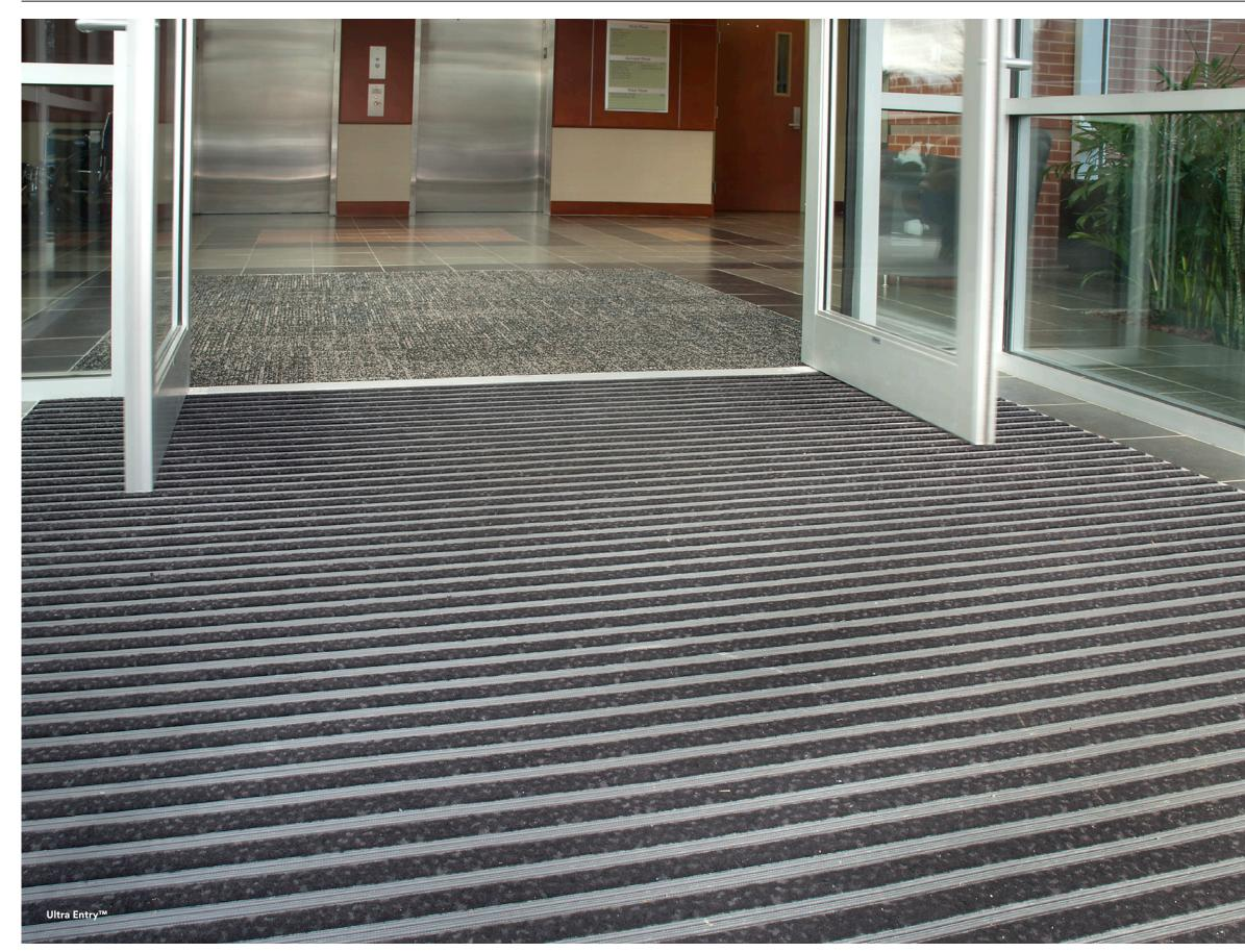
Foot grilles offer many of the benefits of architectural grilles- including promoting positive indoor air quality, removing moisture and debris, and withstanding high foot traffic- without the need for a deep recess.
