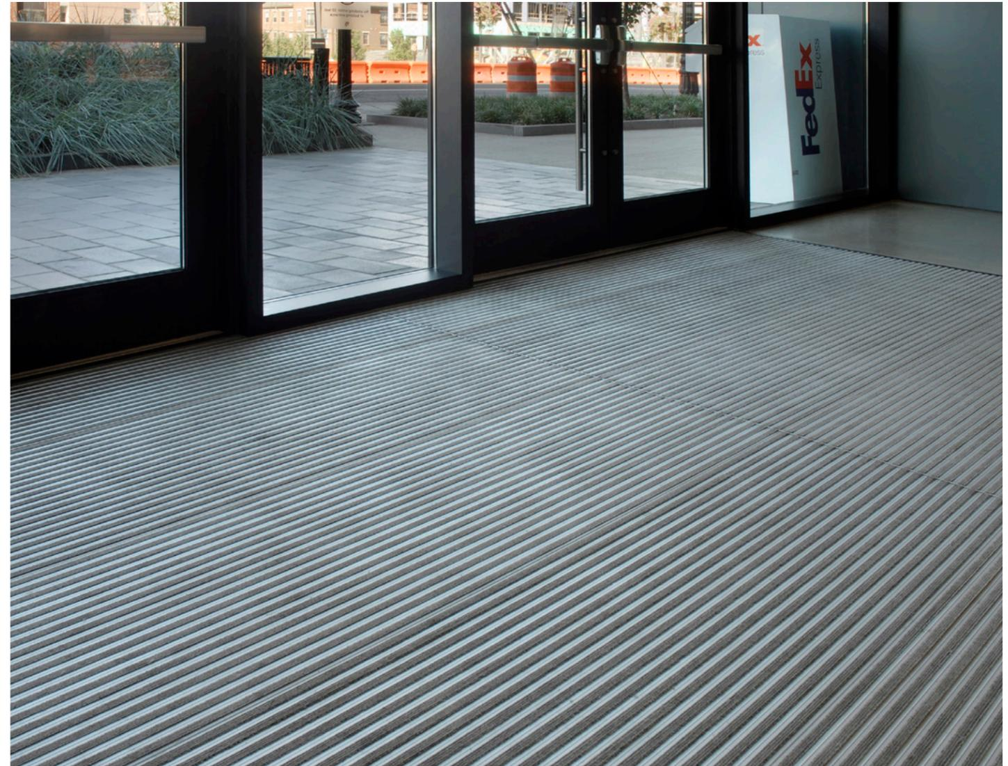
Shallow-recessed system with aluminum and extended matting scraper bars
