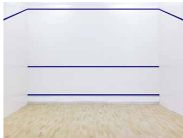
After the Squash Wall Paint application
