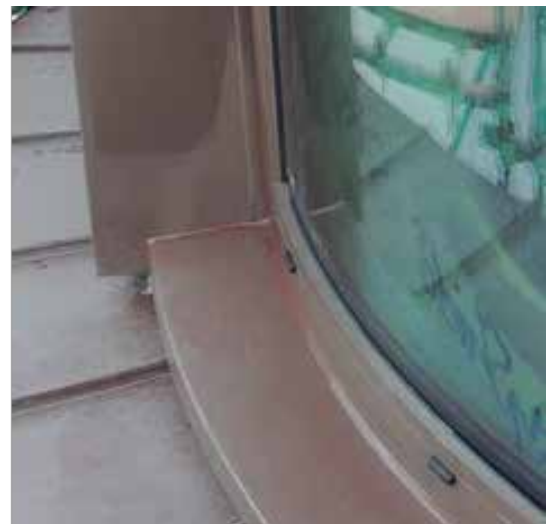
Aluminium window frame sealed against the elZinc Rainbow® Brown sill using brown neutral curing silicone
