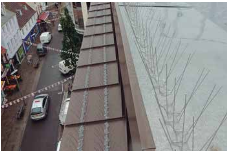
Bird spikes attached using neutral curing silicone
