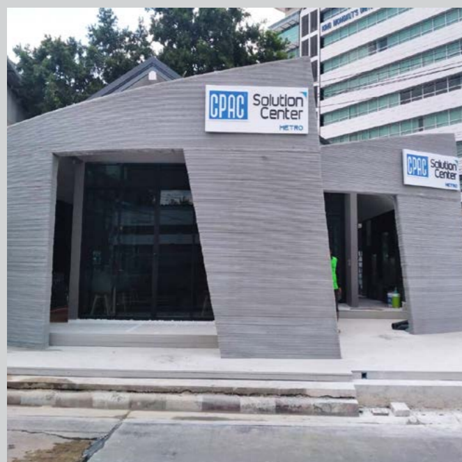
CPAC Solution Center - Metro 3D Concrete Printing Structural Façade
