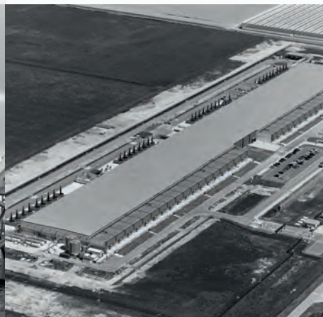
Google Data Center Netherlands
