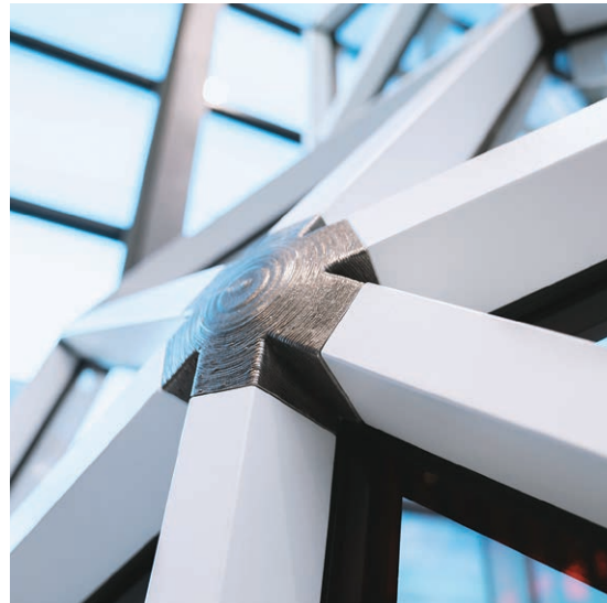
VISS 3 3D printed steel nodes
