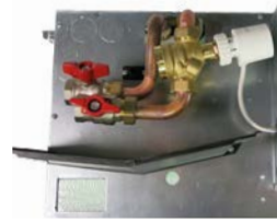
D2B2+DT Pressure independent valve + shut-off valve
