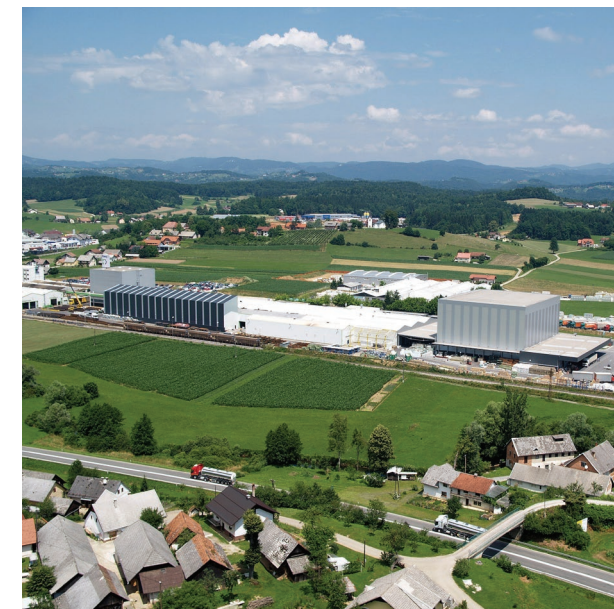
Trimo headquarters and production plant in Slovenia.
