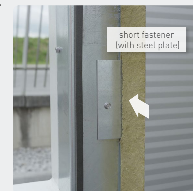
Fig. 3.6: Carrying the vertical load.
