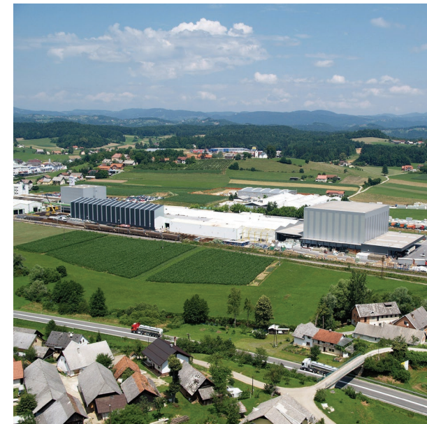
Trimo headquarters and production plant in Slovenia.
