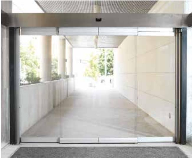
The door functions in normal mode (sliding and automatic). In an emergency, the leaves can be pushed outwards by hand, and automatically retract to the sides to create a large opening for evacuation.
