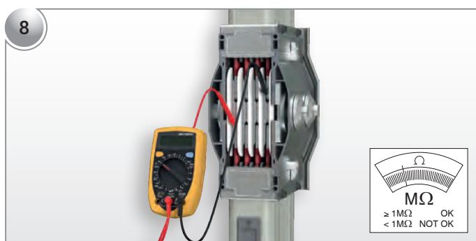
Perform an insulation resistance test between all phases at the installed block joint point.
