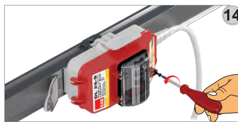
Open the transparent cover of the tap-off box by un-tightening the screw.
