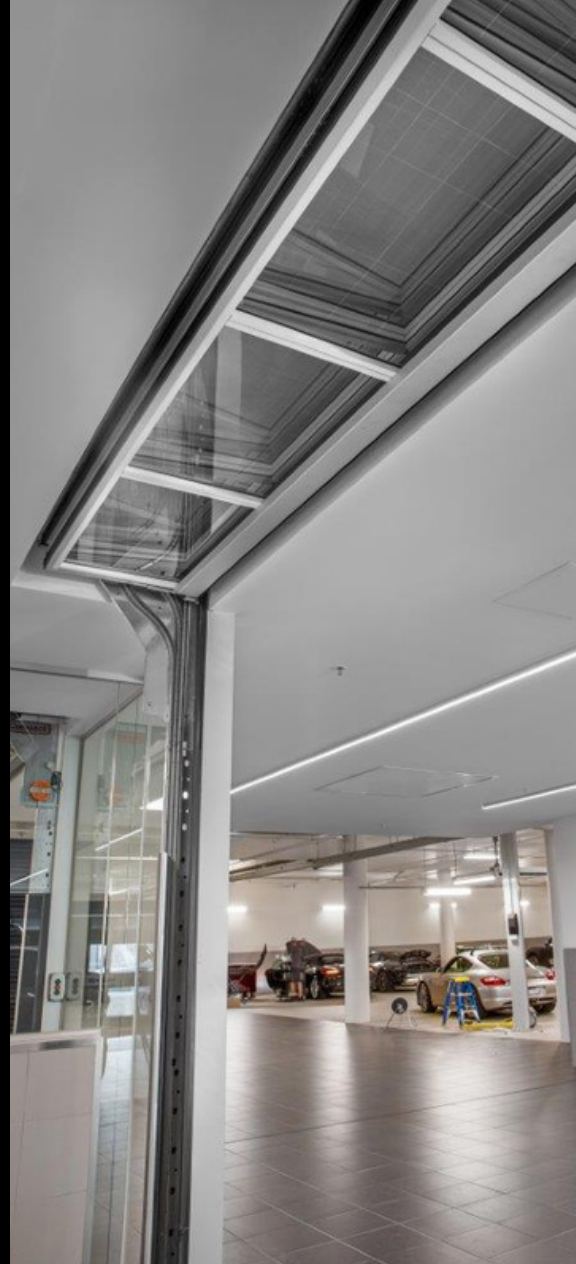
Project: Car dealership, Melbourne, Australia
