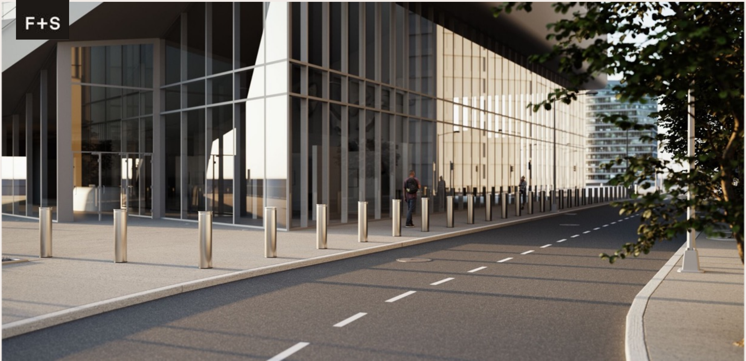
Cyrca Security Bollards
