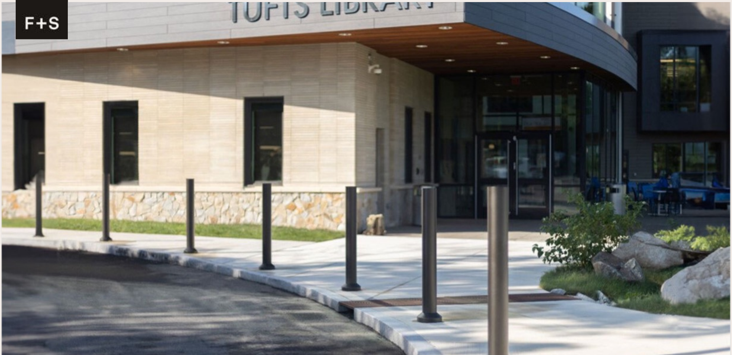
Light Column Security Bollards | Tufts Library
