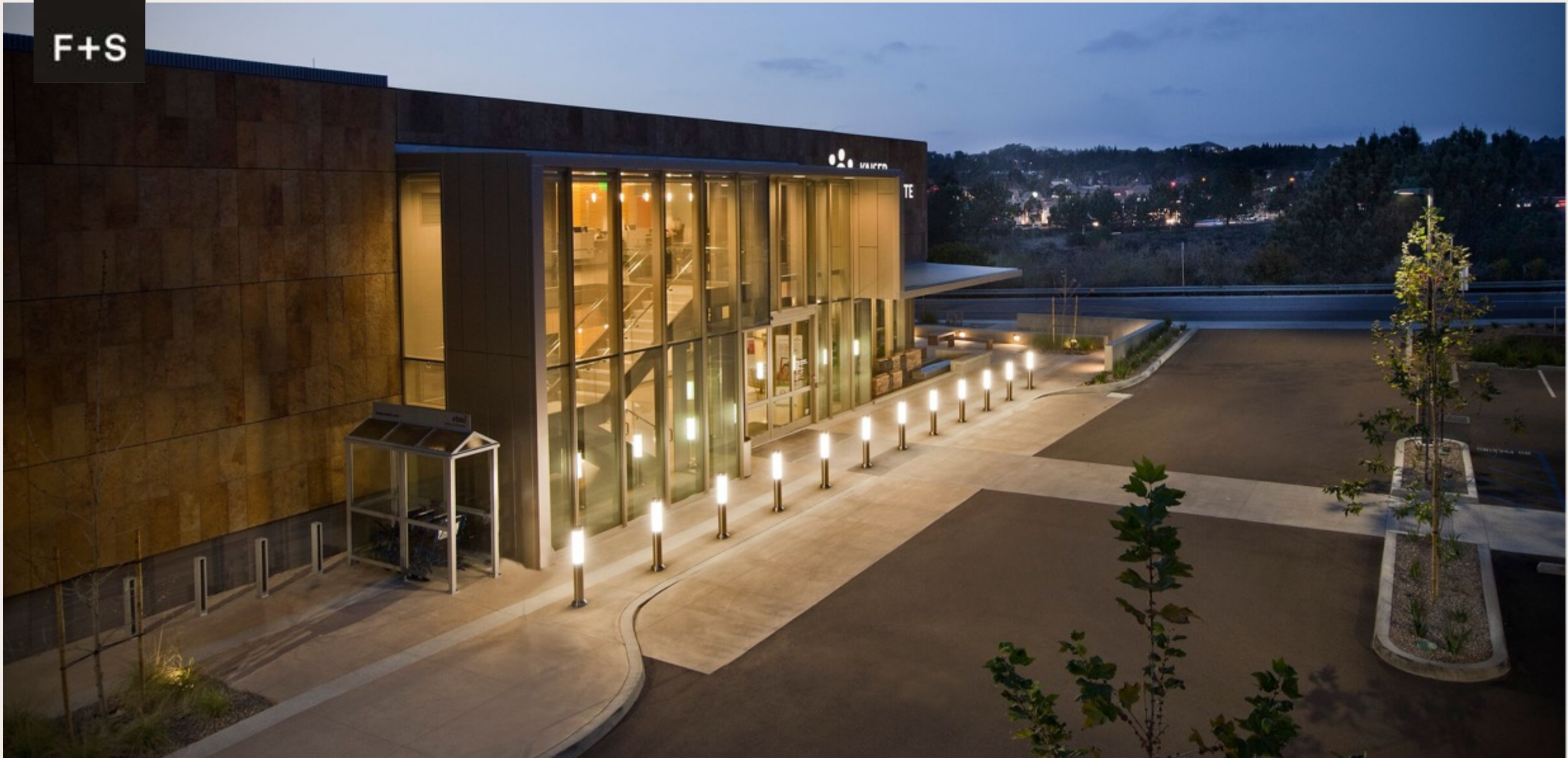
Light Column Bollards | Kaiser Permanente, Carmel Valley Medical Offices
