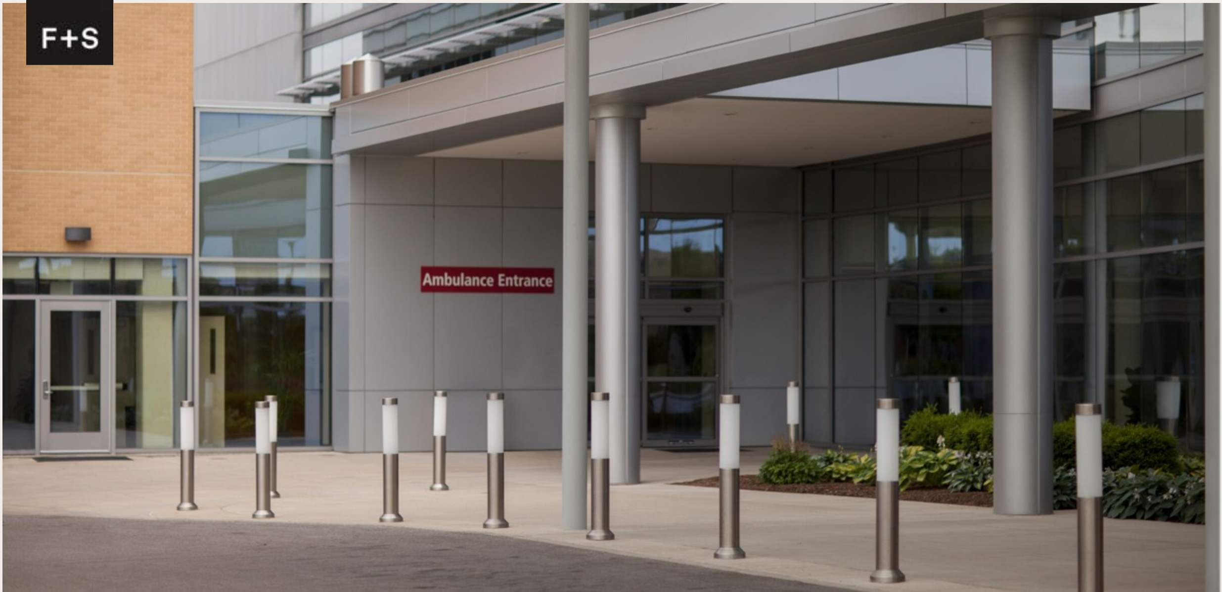
Light Column Bollards | IU Health Neuroscience Center
