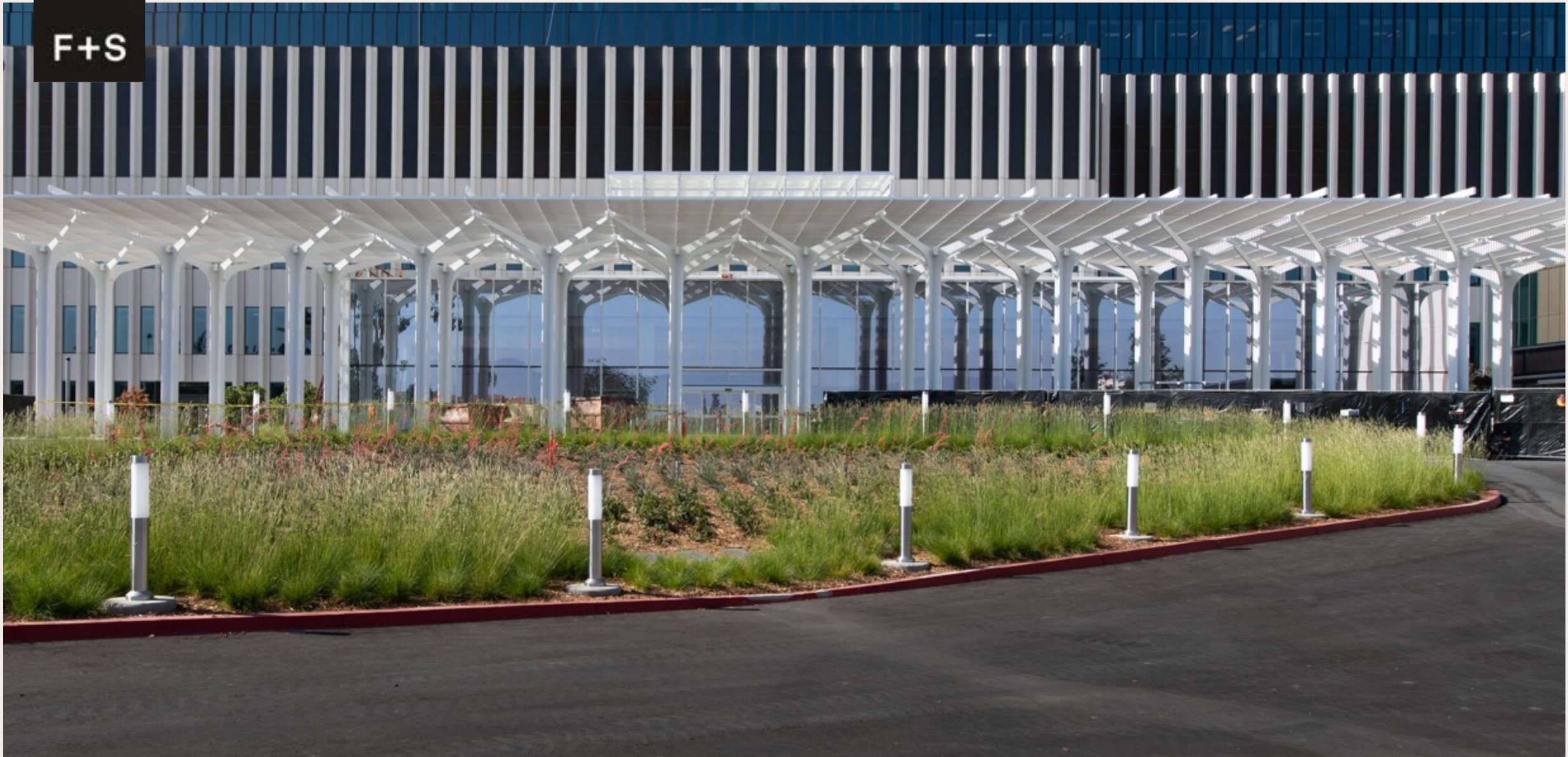
Light Column Bollards | Loma Linda University Health, Dennis and Carol Troesh Medical Campus
