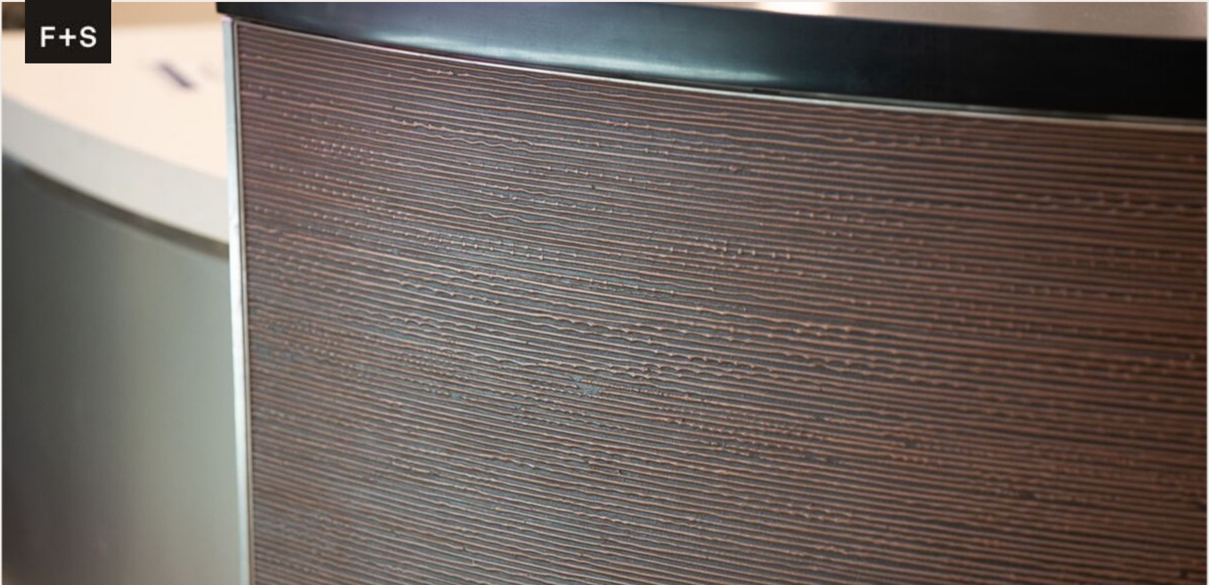
Bonded Metal | Salt Lake City International Airport (SLC)
