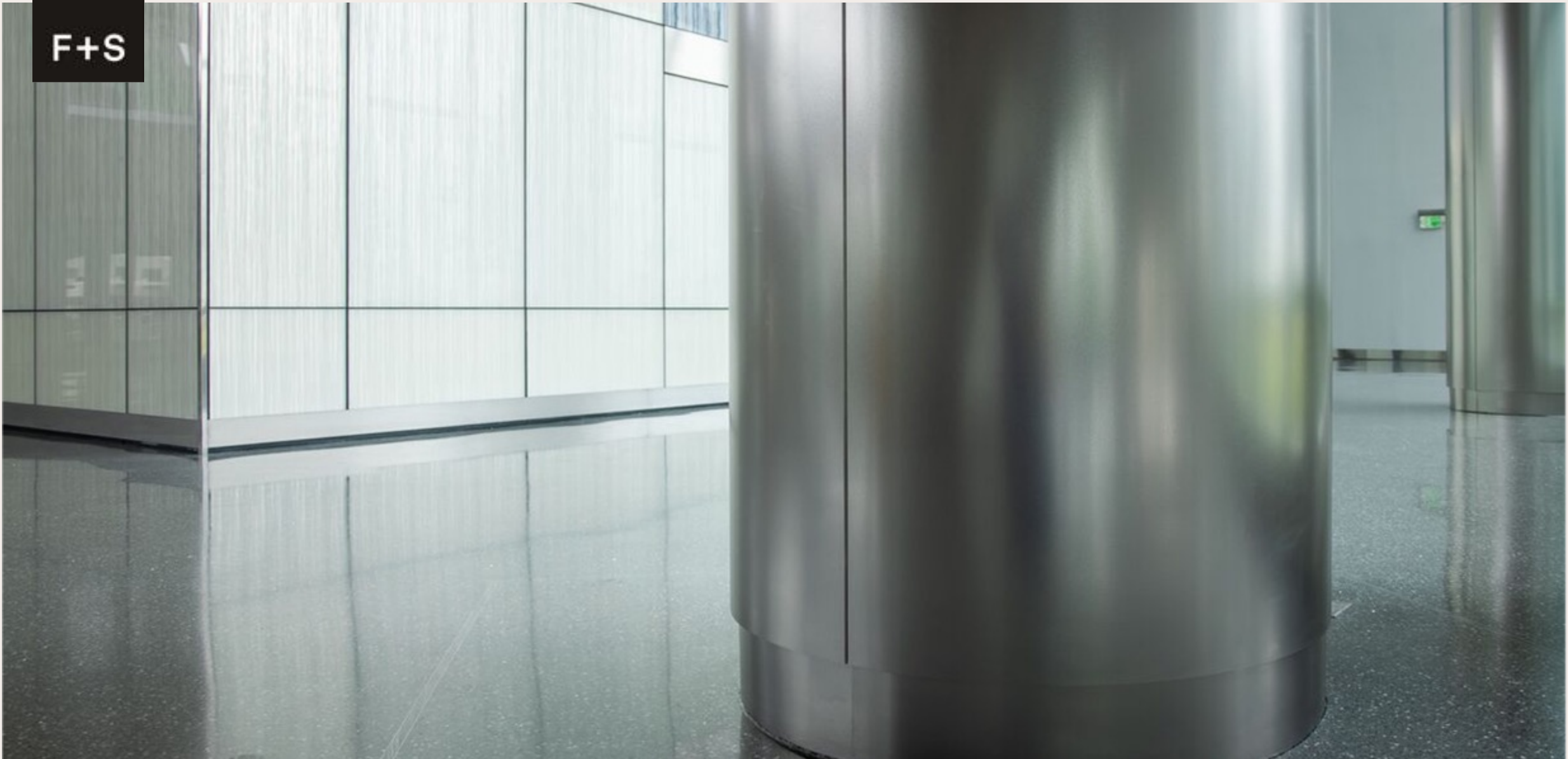
LEVELc Column System, Stainless Steel. LEVELe Wall Panel System, ViviStrata glass | SkyCenter One, Tampa
