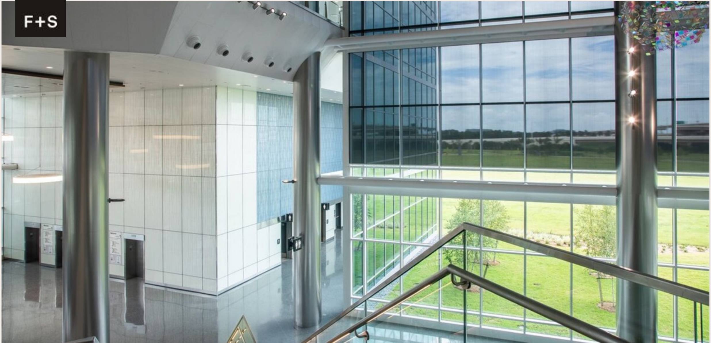
LEVELe Wall Panel System, ViviStrata glass. LEVELc Column System, Stainless Steel | SkyCenter One, Tampa
