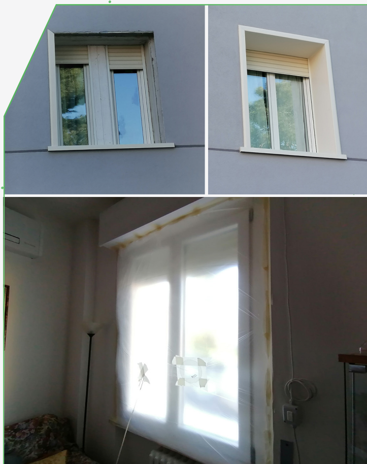
Images of the tests carried out to verify air infiltration.
