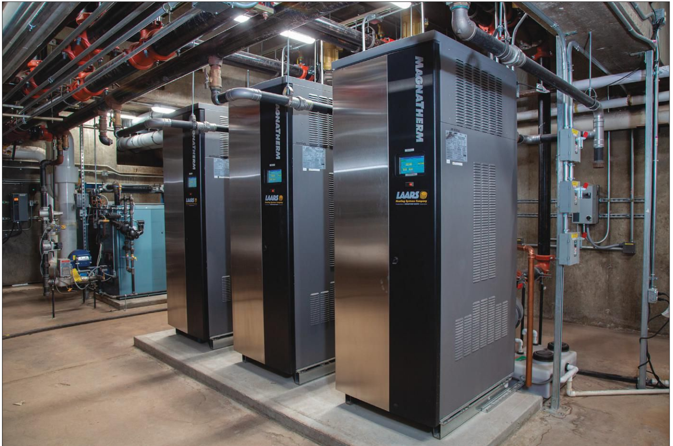
FIGURE 1. A Laars MagnaTherm® HTD Boiler installation. Images courtesy of Laars Heating Systems Company
