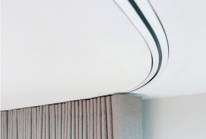
Trackrim® Curved Section finished installation.
