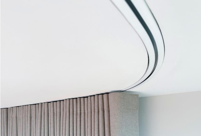
Trackrim® Curved Section finished installation.
