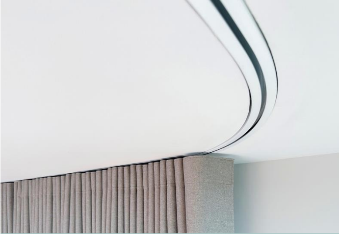
Tracktrim® Curved Section finished installation.
